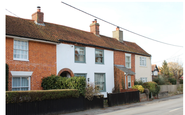
Figure 43 The group value of terraces is particularly vulnerable to incremental change
