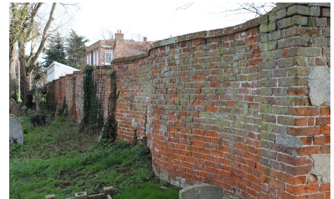
Figure 31 The listed Crinkle-Crankle Wall, which gets its name from its S shape, bendy form
