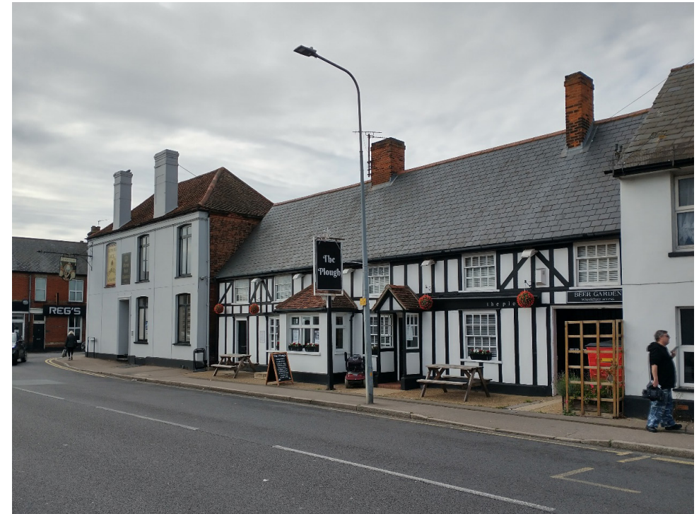
Figure 2 The Grade II listed Queen's Head former public house and The Plough on North Road
