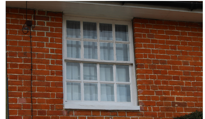
Figure 30 Example of a timber sash window
