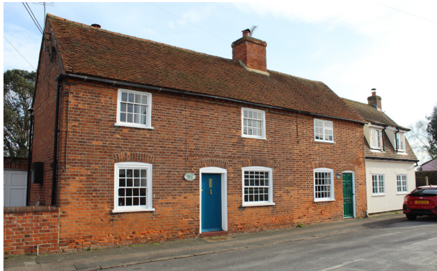
Figure 25 An example of a brick and rendered building with timber windows and doors
