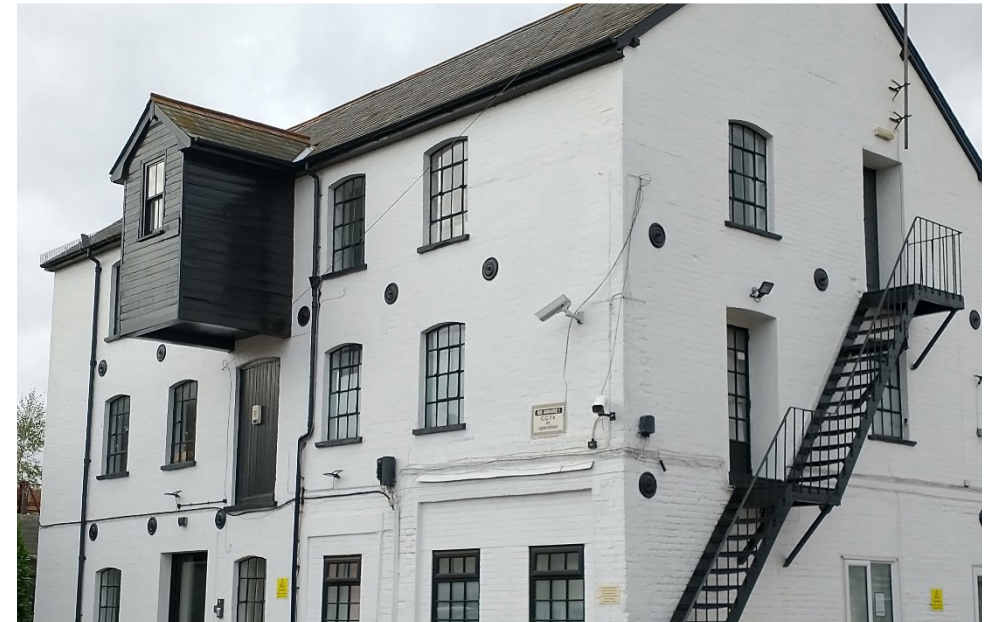
Figure 31 The Mill on Old Road in the setting of the Conservation Area
