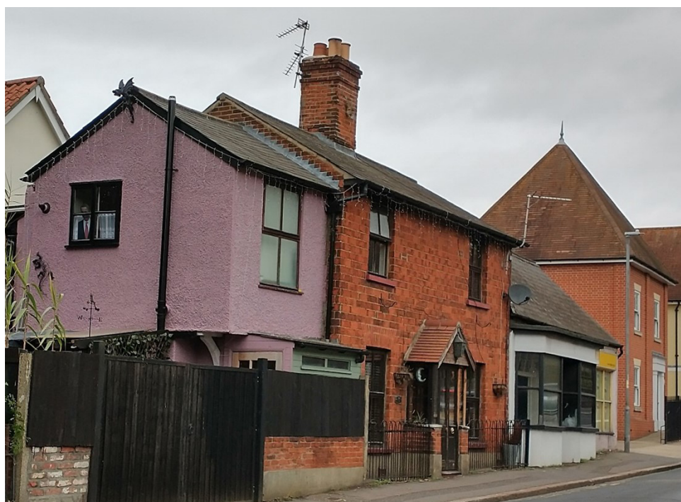
Figure 24 Number 395 Old Road in red brick laid in Rat Trap bond, with numbers 399 and 397 to the north
