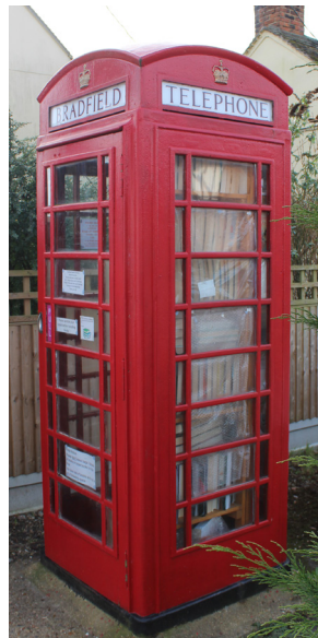
Figure 34 Listed K6 Telephone Box
