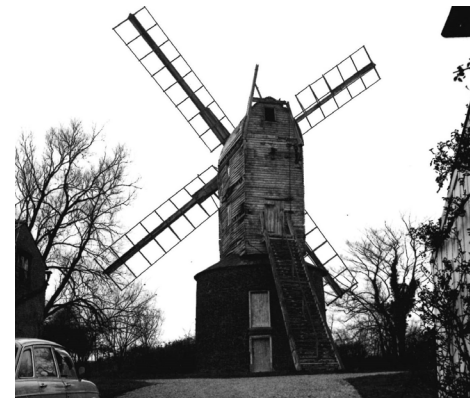
Figure 15 Ramsey Windmill in 1974, viewed from the south. Note deteriorated state of weatherboarding and access stairs
